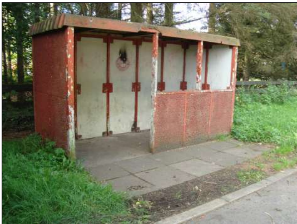
Plate 1: RCP Shelter at Stranocum (Fivey Rd) in poor condition and subject to repeated anti social behavior including graffiti, litter and drinking.
